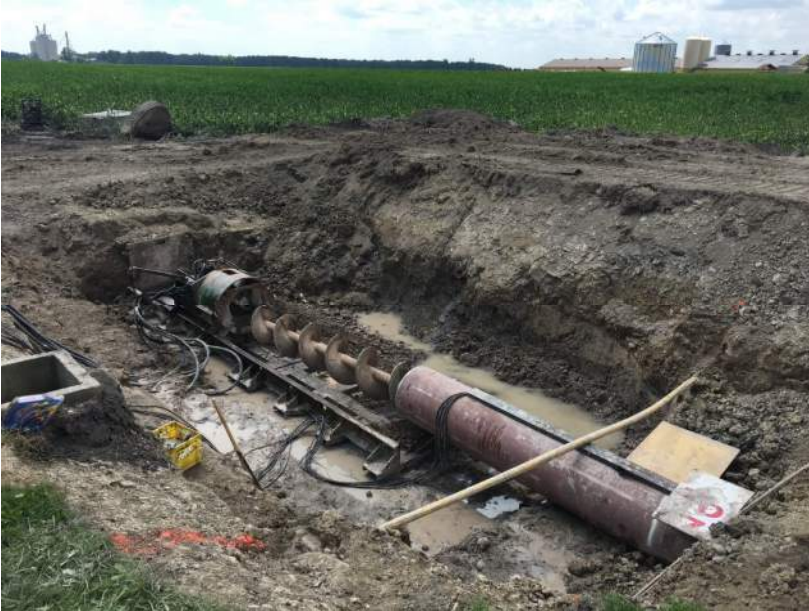
Jack and Bore Pipe Installation
