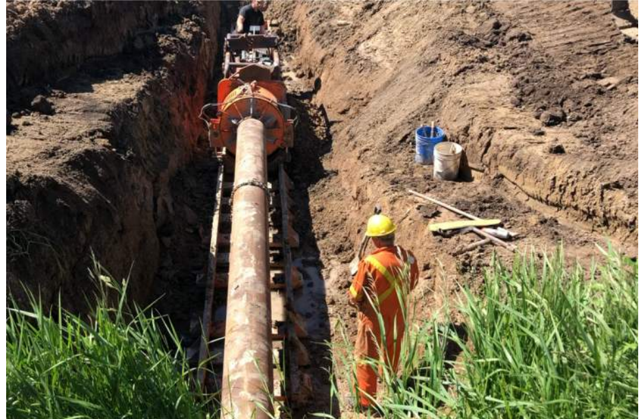
Video of Jack and Bore Pipe Installation
