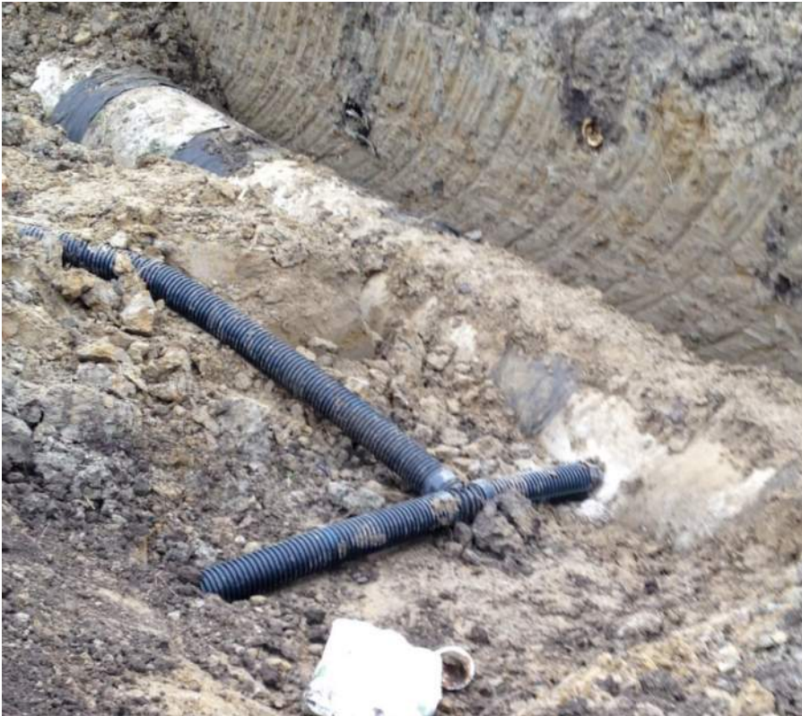
Tile connection into a Municipal Drain
