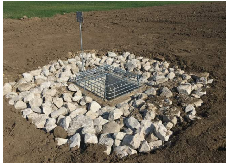
Example of a flat top catchbasin complete with rip-rap erosion protection
