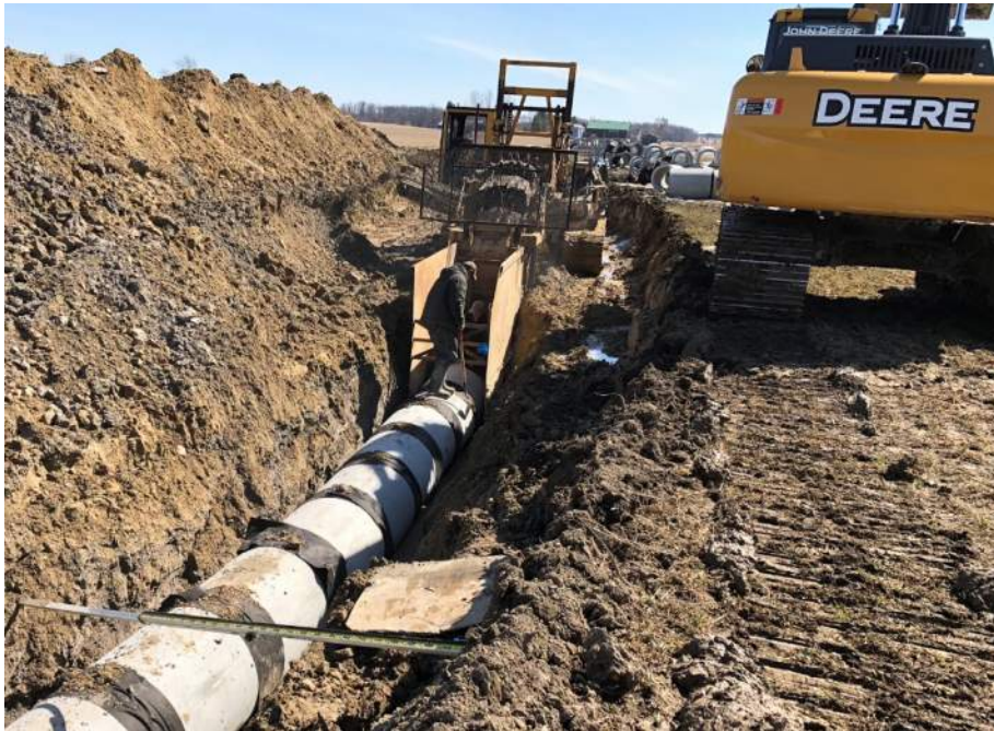
Example of a Municipal Drain Being Installed via Wheel Trencher
