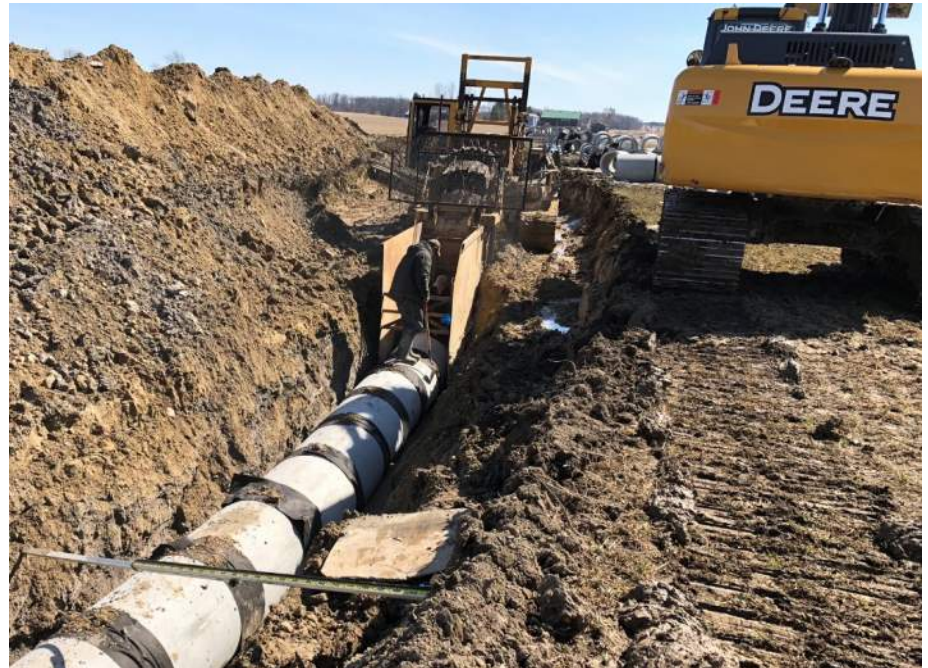
Example of a Municipal Drain Being Installed via Wheel Trencher
