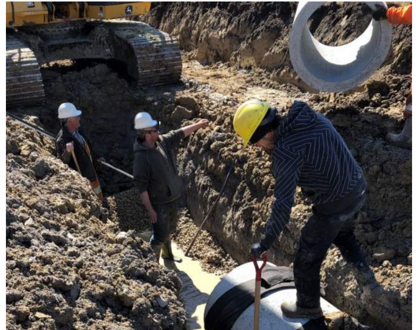
Example of a Municipal Drain Being Installed via an Excavator on Stone Bedding
