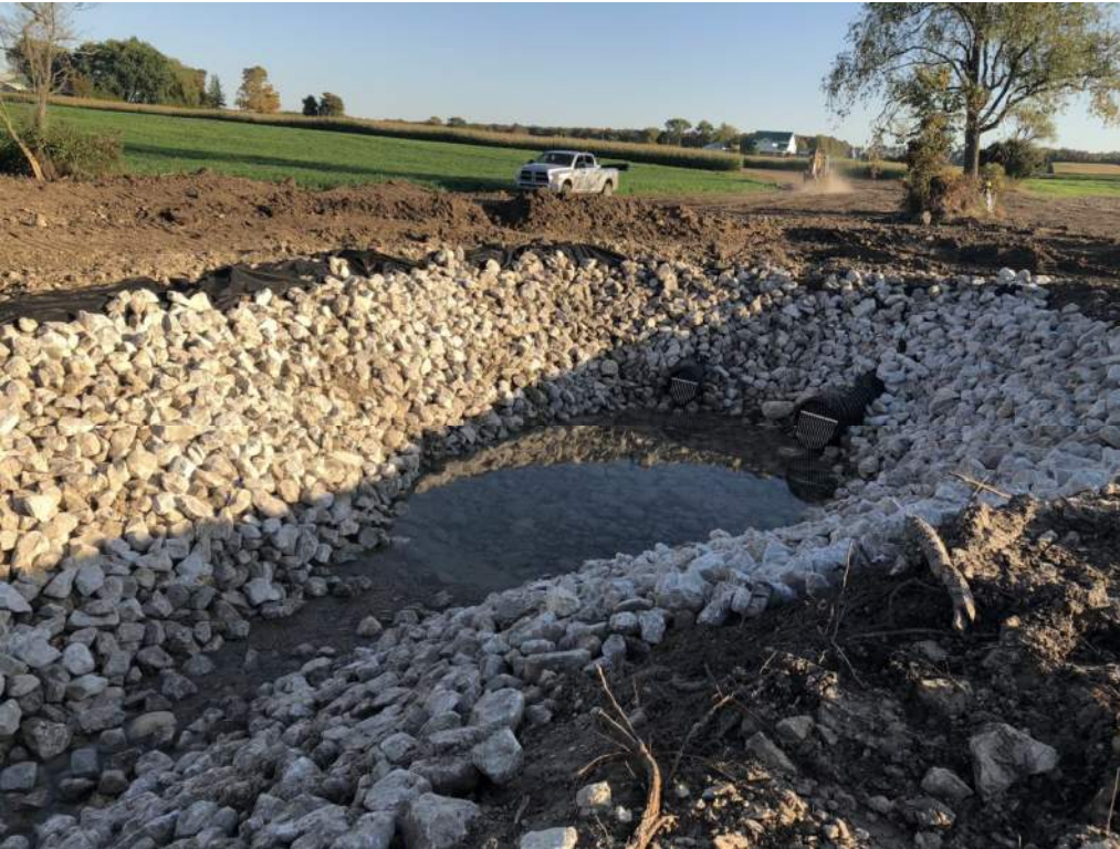
Newly Constructed Stilling Basin
