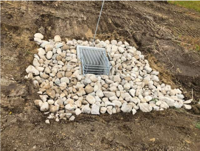
Dich inlet catchbasin complete with rip-rap erosion protection
