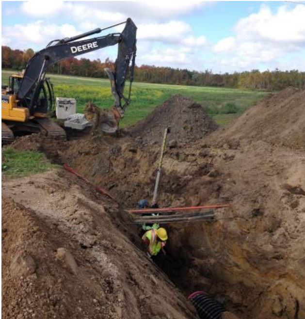
Open Cut Installation Method
